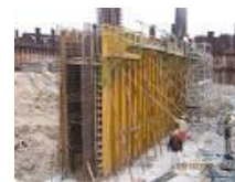
Wall formwork
