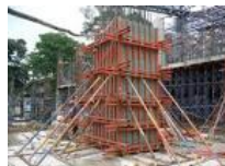
Column formwork
