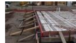
Slab formwork
