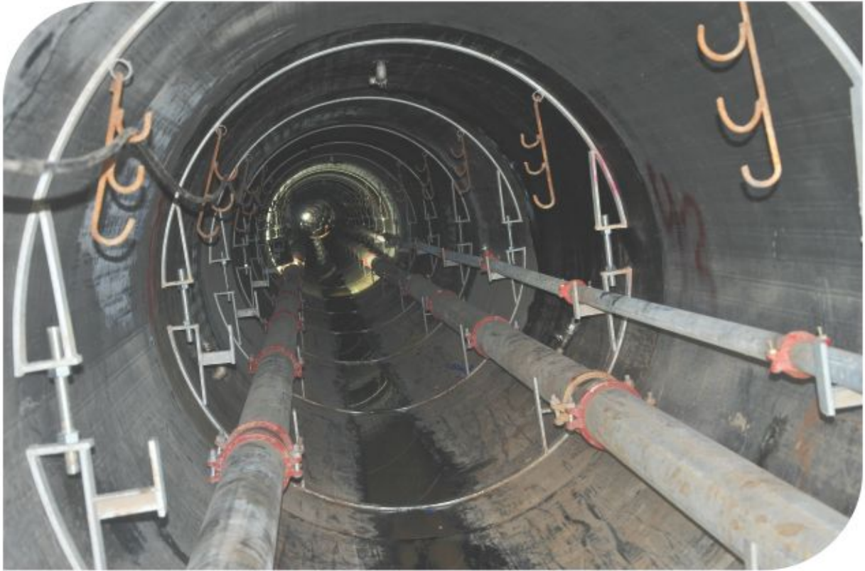
DJB Micro Tunneling Project
